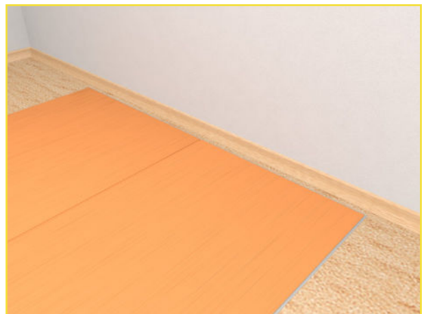
Fig.22: Laying out the screen material
